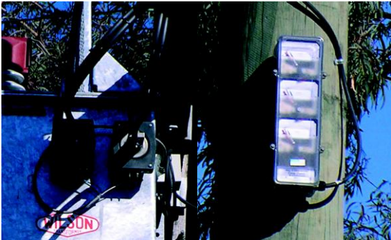
Type 73D Maximum Demand Indicator mounted on pole adjacent transformer.
